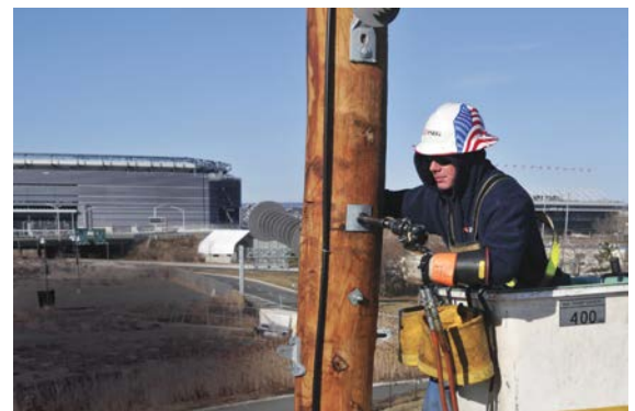
A PSE&G lineworker prepares to install a new 69 kV line. The utility's plans to upgrade infrastructure after Sandy have been scaled back due to concerns about cost.
