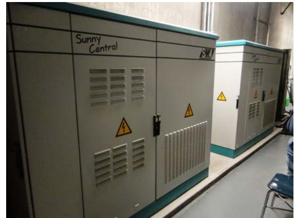
Two SMA Sunny Central commercial inverters help create a solar/diesel microgrid for an emergency shelter in Bayonne, New Jersey.
