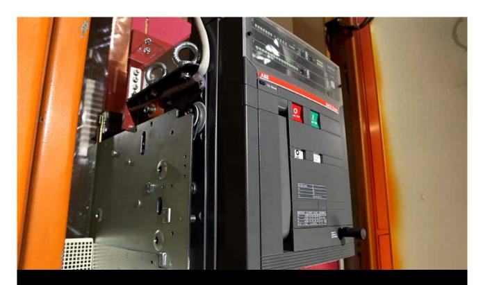
Retrofitting kit New Emax Direct Replacement of Megamax and Novomax
