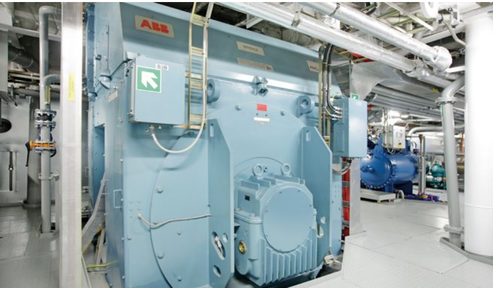
High voltage marine generator
