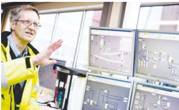
ABB's System 800xA provides precise process control, allowing the plant to be operated close to its safety margins.
