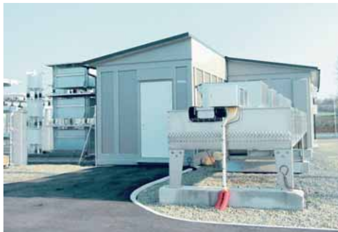
Outdoor substation module for mainline railway
