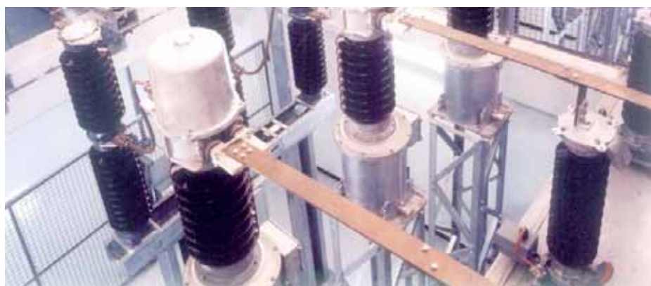
66/22 kV air insulated - indoor type substation
