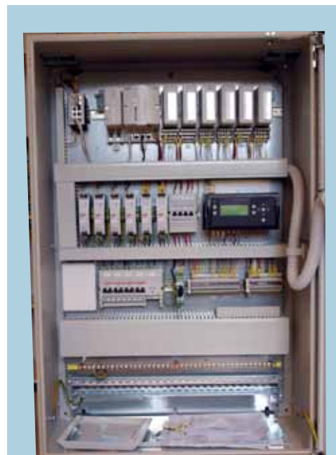
Figure 4: Up to 75% of a stand-alone PMS cabinet is occupied by power and external interface components which can be eliminated with careful integration
