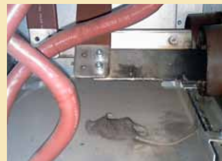
Figure 3: A rodent causing short circuit in an MV switchboard. Due to installed arc protection system, only minor damages were caused.
