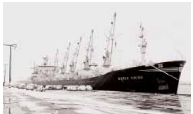
The "Viking Norse" was equipped with six 8-ton, electro-hydraulic, programmable deck cranes (late 1970s).
