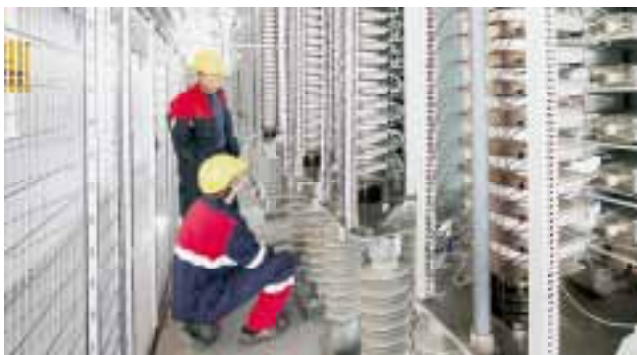
FACTS installation to support increasing electricity demand in Norway, 2009. FACTS technologies can enhance the security, capacity and flexibility of transmission systems.
