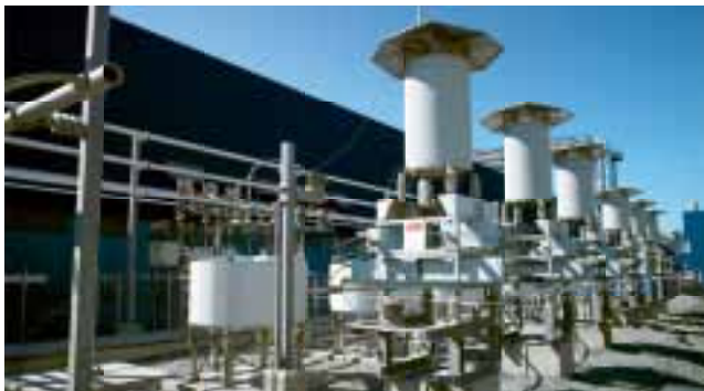
A FACTS installation in Finland, 2005, stabilizing voltage and current fluctuations in Finland, 2006. The technology helps to counteract interference with local power networks that cause problems such as lighting flicker.
