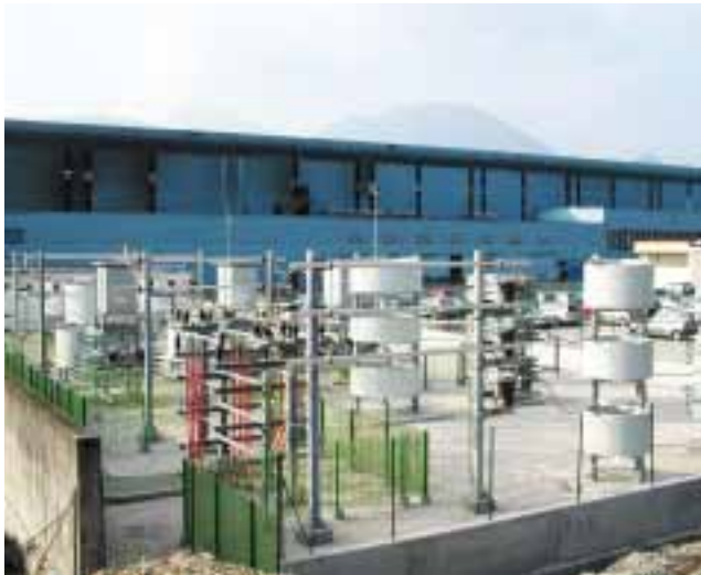
A FACTS installation at a steel mill in Italy, 2002. By improving the power quality in such plants, FACTS technology can raise productivity by several percentage points.
