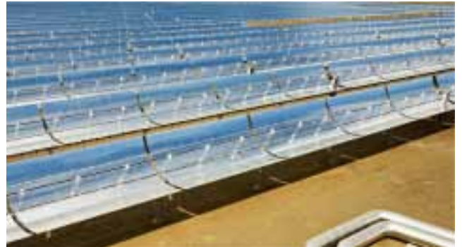
System 800xA is used to control parabolic mirrors in Europe's largest thermal solar power plant, Andasol, in southern Spain. Tracking the sun's movement across the sky ensures maximum productivity.
