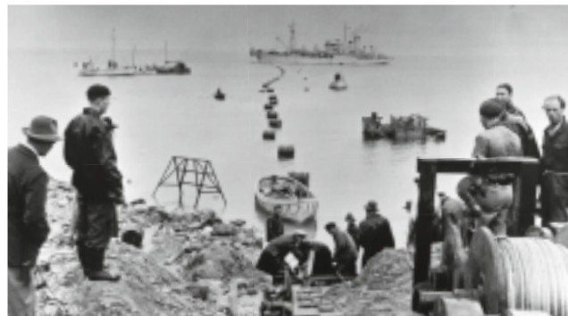
Pulling the Gotland cable ashore in 1950. The power link connected the island to Sweden's mainland power grid, supporting the development of the island's economy.
