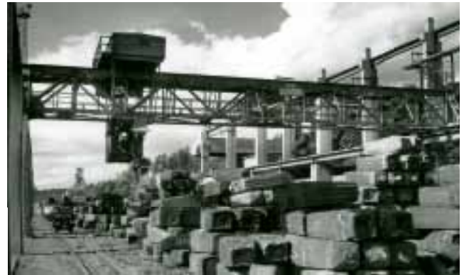
An Asea magnetic gantry crane at Fagersta Bruks AB, Sweden. The crane has a 30m span and lifting capacity of up to 12 tons (1950s).
