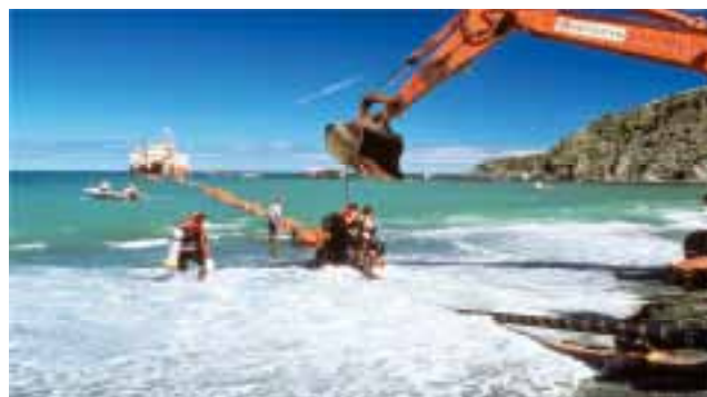
Laying cables for the New Zealand interisland link across the Cook Strait, 1985. The link delivers hydropower from the South Island to centers of demand in the north.
