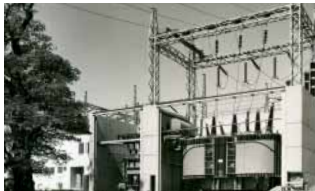
In 1942, Asea delivered what was then the world's largest transformer (120 MVA, 220 kV) to the Värtan substation in Stockholm.
