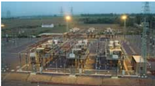
FACTS installations at Raipur in India, enabling power to be transferred from India's eastern power grid to the west and south of the country.
