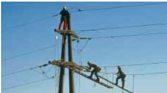
Engineers integrate fiber-optic cables into existing transmission lines for Swiss utility EKZ in 2006. ABB's communication equipment is used world wide to transmit voice, data, and protection signals on high-voltage lines.
