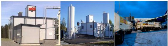
The Etanolix® technology performs these two processes simultaneously and in situ, or close to the sources of the raw material (i.e. biowaste or food waste). This means less operational energy consumption and less transportation or landfill costs incurred by biowaste producers.
