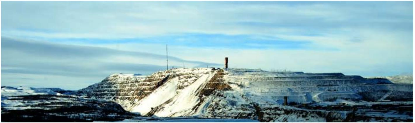
When LKAB increases the production from 26 to 33 million tonnes of crude ore per year, hoist capacity is of vital importance. The first measure taken was to upgrade the four sub-vertical level hoists from DC to AC-technology. The second is to install a fifth double skip hoist on this level in order to start operating the new production level at -1365 m. The present four hoists will continue with the -1045 production level until production on this level ceases.
