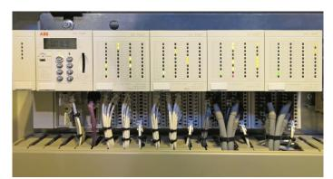
The Freelance controller AC 700F with S700 direct I/O
