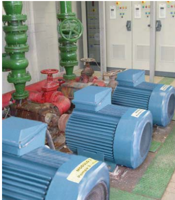
The switch room of the Fonte La Penna pumping station in Sezze Latina, near Rome, had its outdated control system replaced with low voltage AC drives, resulting in better operation and reduced energy bills.
