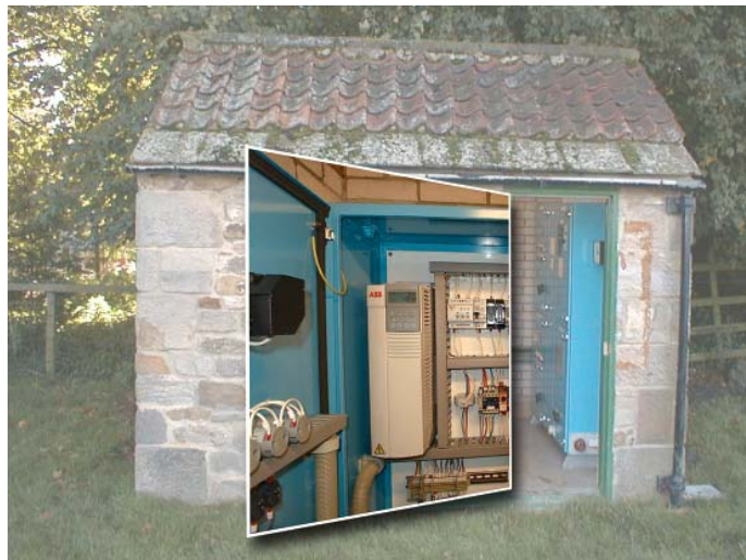
An ABB drive is helping Northumbrian Water to save up to 50,000 pounds by running its 3-phase equipment from a 2-phase supply.
