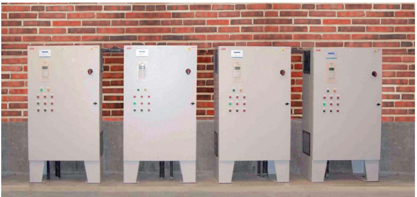
ABB industrial drives are installed on four 93 kW pump motors to improve performance.
