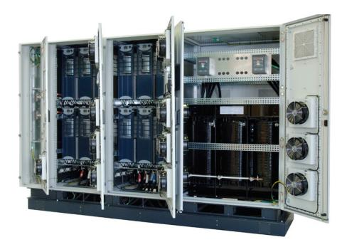
The PCS100 SFC is a proven, efficient and effective power system that is specifically designed to interconnect incompatible networks. The PCS100 SFC units installed replaced former technology to give a highly reliable system that is a more flexible, efficient, and cost competitive approach to supplying the frequency and voltage neccessary. This particular application has been designed to supply power from the platform to the vessel, avoiding operation of its onboard diesel enerators...
