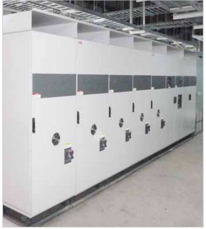
A PCS100 UPS-I installation with ultra capacitor storage in a semiconductor facility
