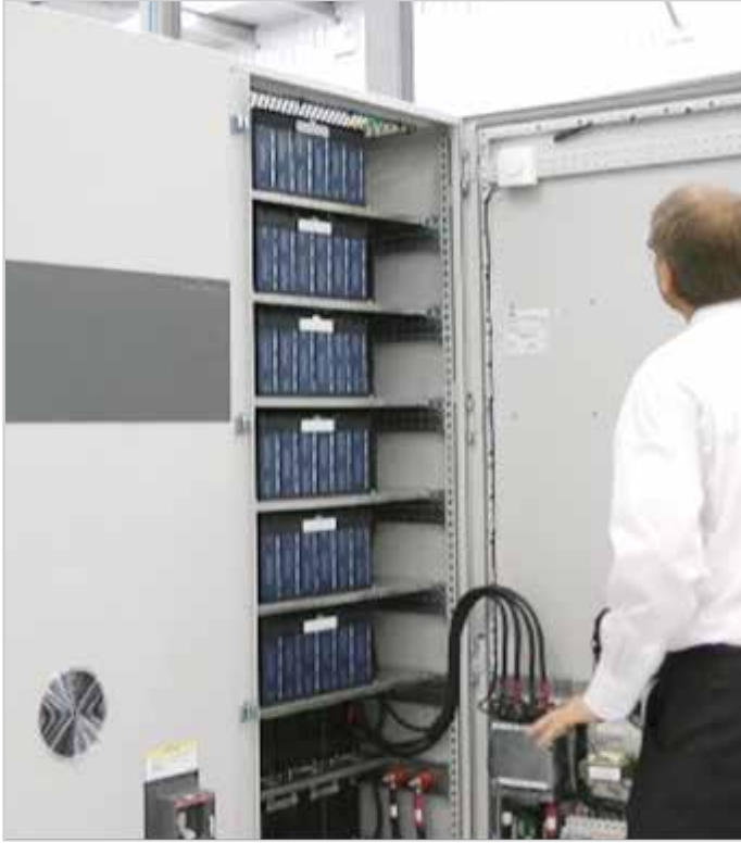
LS Mtron ultra capacitor module installed in PCS100 UPS-I Industrial UPSs
