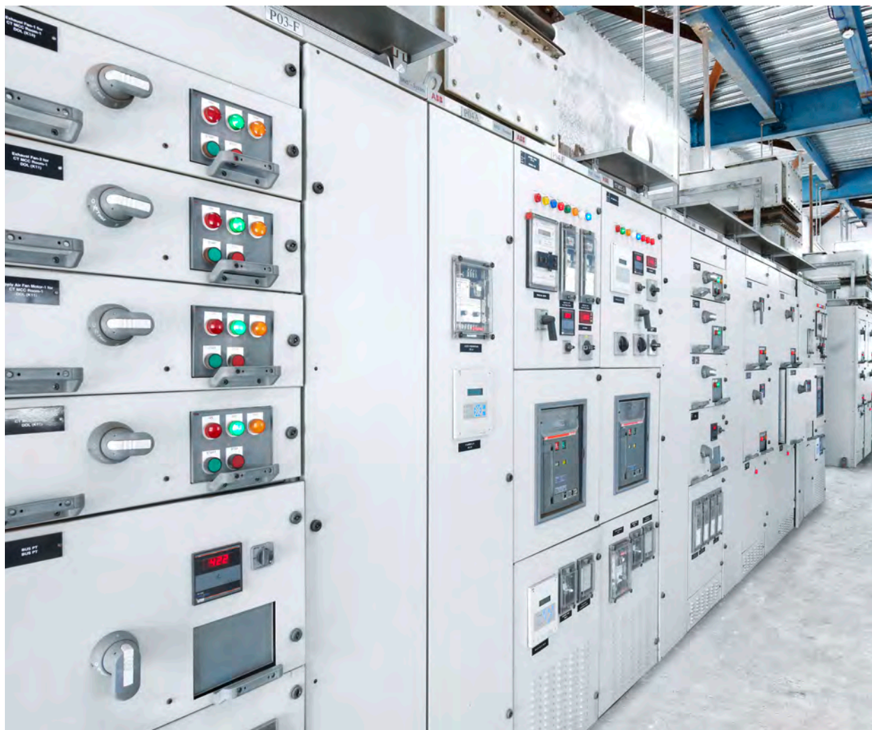
Figure 2.15: Example of a main distribution switchboard
