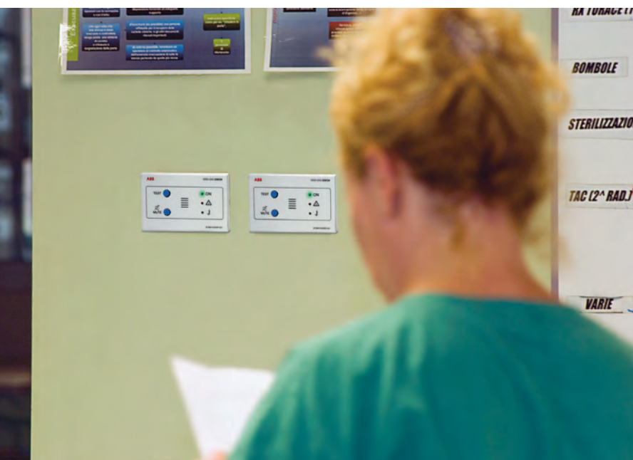
Figure 3.8: QSD remote signalling panels allow medical personnel to be immediately aware of malfunction situations
