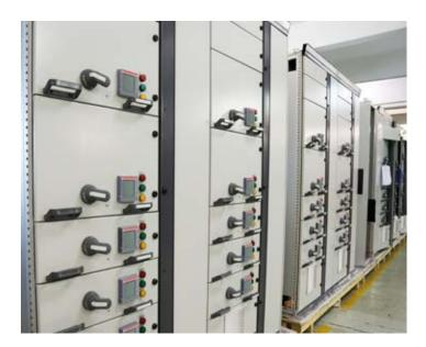
The available module types have typical characteristics as shown in the graphic above. Where high process availability is essential and minimal time is required for module exchange the with drawable solution has proved to be the definitive choice.
