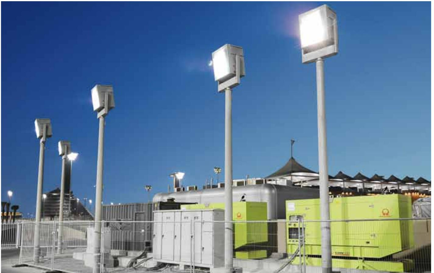
Pramac supplied 44 electricity generators for the lighting system of the Abu Dhabi Formula 1 Grand Prix track. Each one has electrical power from 250 kW to 370 kW and is able to supply enough power to light more than 4,000 flats. Pramac generators are equipped with special anti-sand filters able to prevent any potential blackouts caused by desert sand storms.
