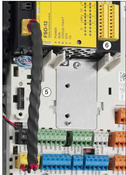
7. Connect the power supply wires to the FSO terminal X112. Use a tightening torque of 0.24 Nm (2.1 lbf·in) for the FSO terminals. Use proper cable strain relief. See also section [Power supply connection/cables](#) on page 231.
