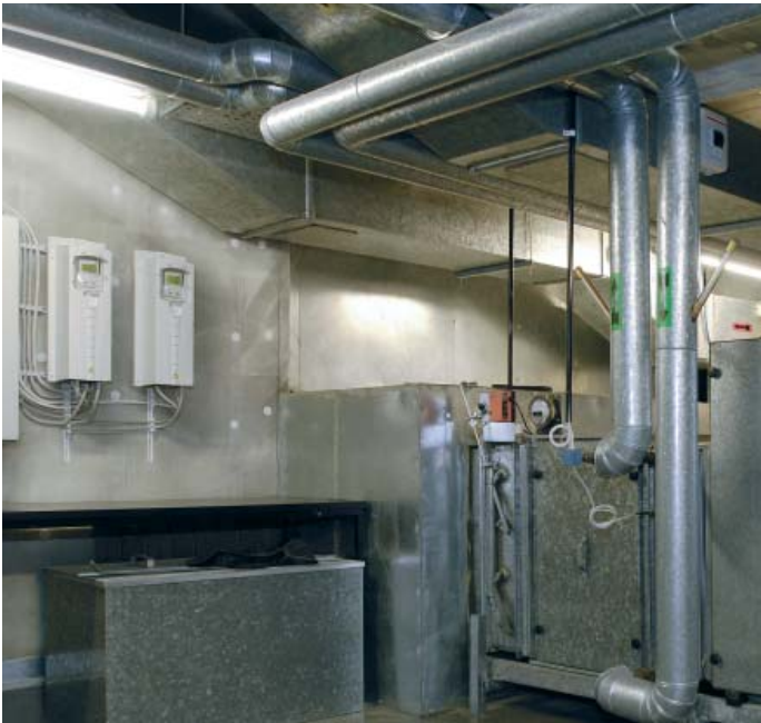
The Airwecare solution uses ABB standard drives for HVAC, controlling new high efficiency Eff1 ABB motors, which in turn drive the supply and return fans.
