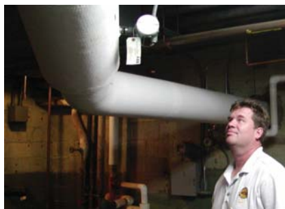
Pat Dillon, electrical and control technician, views a new swirl flowmeter.
