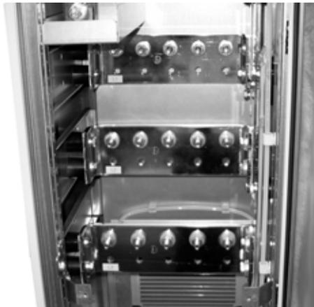
*Grid cable connection terminals L1, L2, L3*
