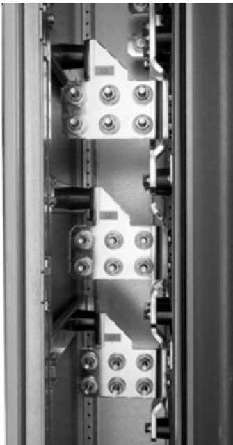
*Grid cable connection terminals L1, L2, L3*
