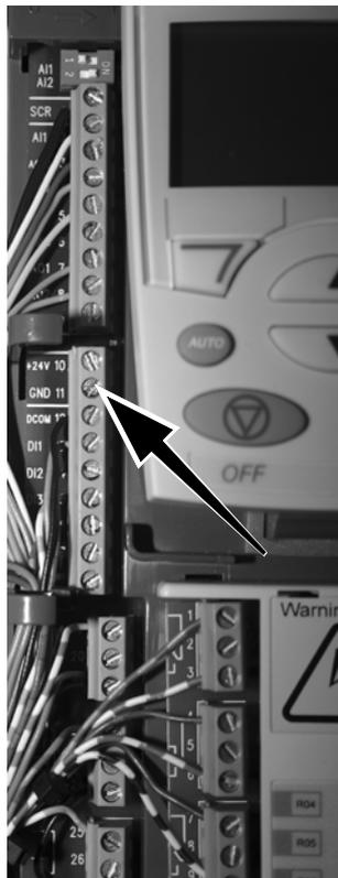
4. Mount the power connector to the drive's internal 24 V DC connection on terminals 10 and 11.
