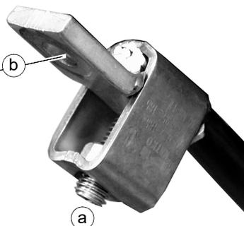
**a.** Connect the cable to the terminal.
