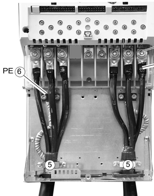
Remove the screw terminals. Fasten the cable lugs to the remaining bolts with M10 nuts.
