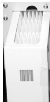
4. Check the cleanliness of the cabinet. Clean the interior of the cabinet if necessary using a soft brush and a vacuum cleaner.
