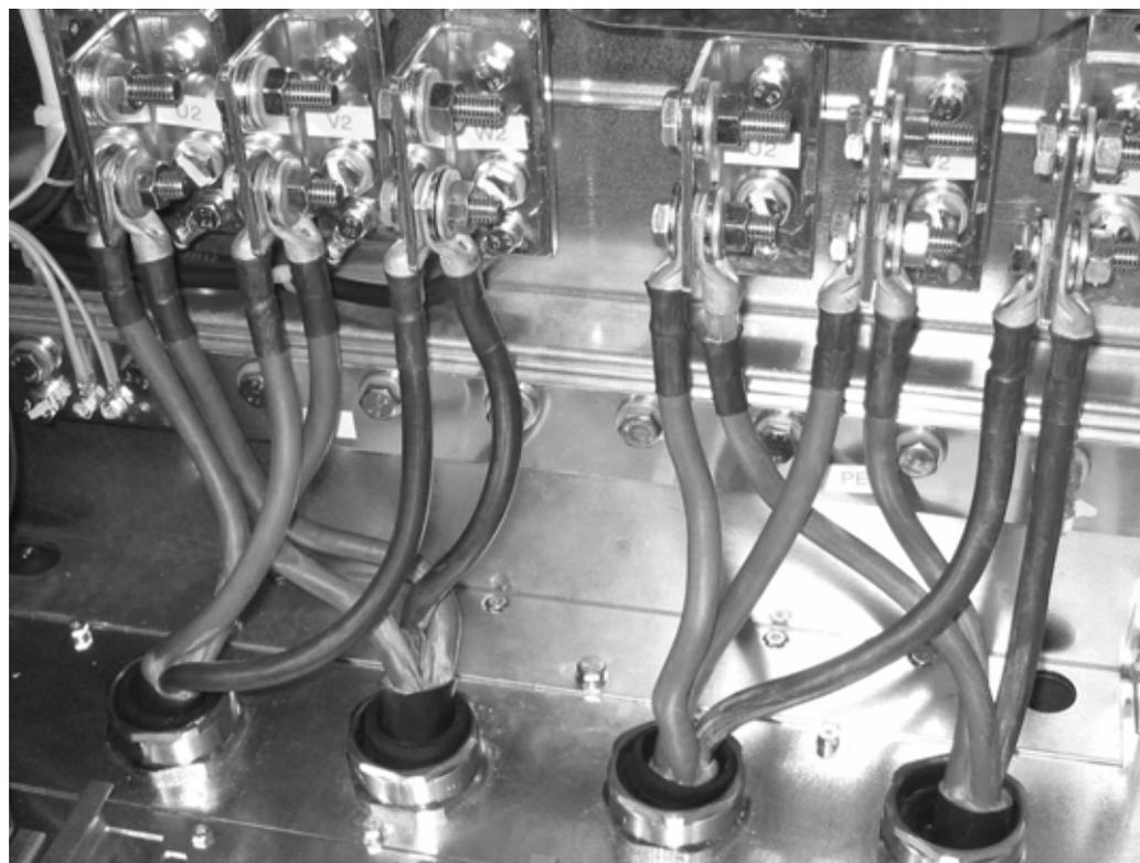
All rotor-side converter modules (two are shown below) are to be connected in parallel. It is recommended that the cabling from all rotor-side converter modules to the rotor is physically identical considering cable type, cross-sectional area, and length. Jumping the output cables from one rotor-side converter to another (and then to the rotor) is also possible, but not recommended.
