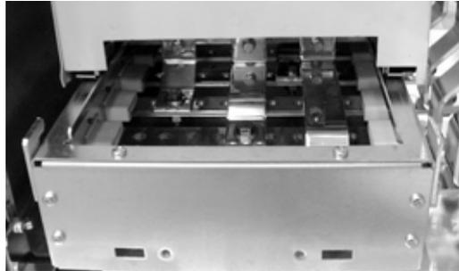
*The module is slid in on the pedestal rails (view from back, the back plate of the cabinet removed)*
