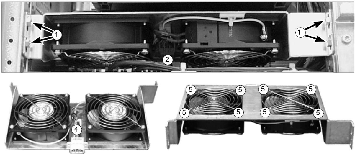
**Replacing the additional cabinet fan (frame sizes R7 and R8 only with IP22 and IP42 when cabling: bottom entry/exit)**
